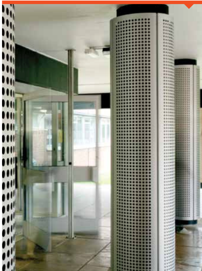
Exeter University: GA Perforated Column Casings with Shadow Gaps.
