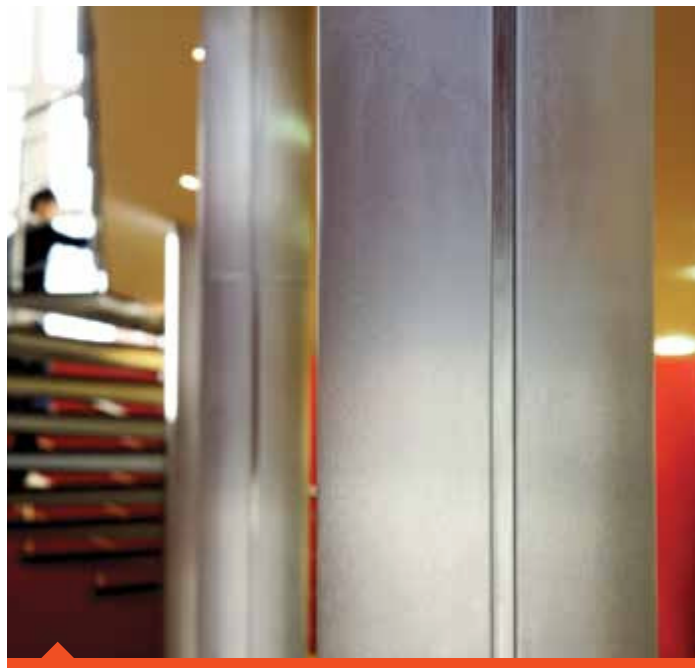
Portsmouth College: Satin brushed column casings with shadow gap infills
