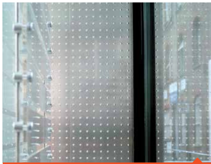
Carlisle Street Lobby: GA Impressional Wall Cladding
